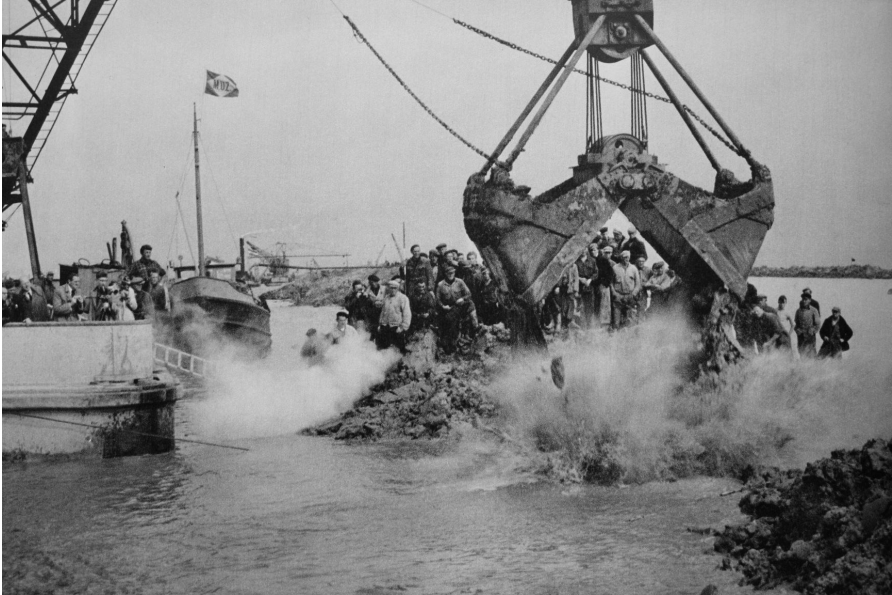
Figure 4.1 Closing the dykes during the draining of the Eastern Flevoland polder, 1956
